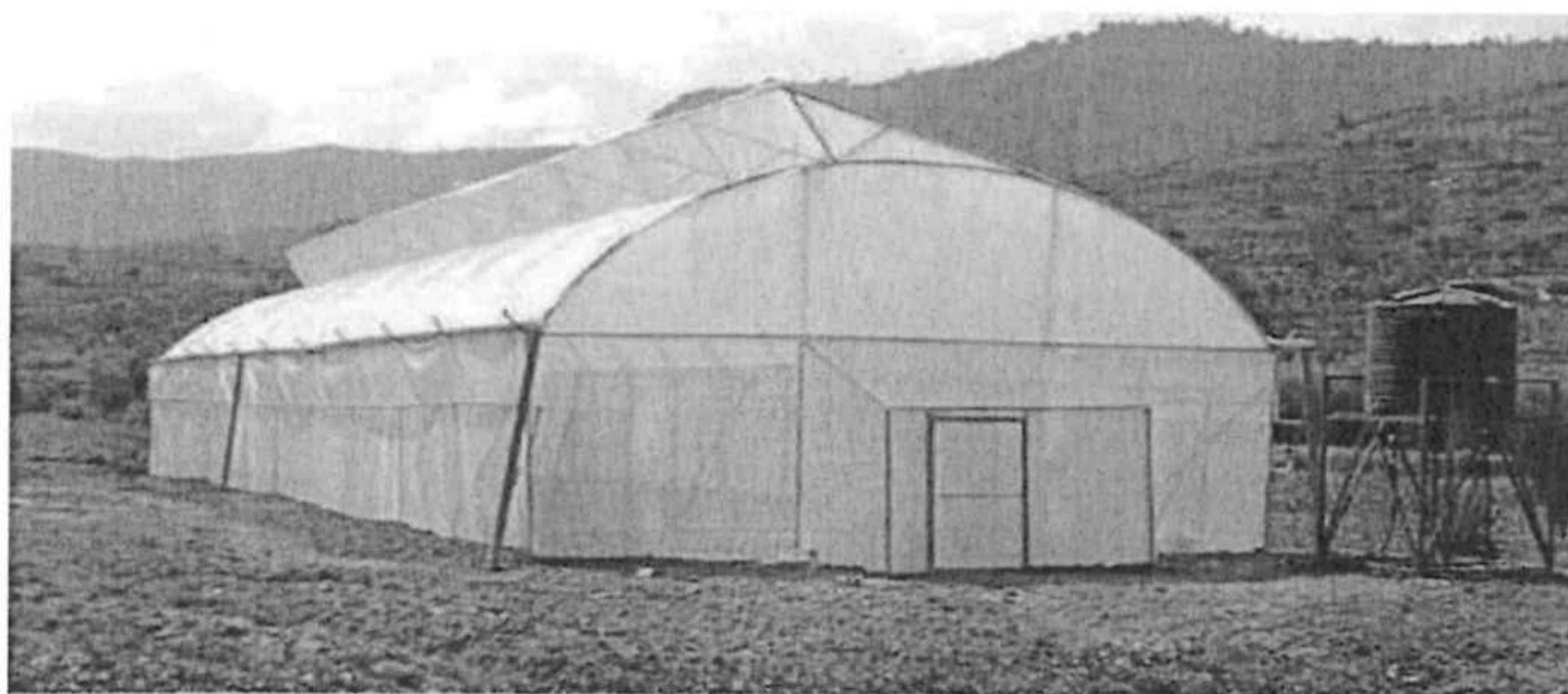
Picture: 8MX30M installed greenhouses
